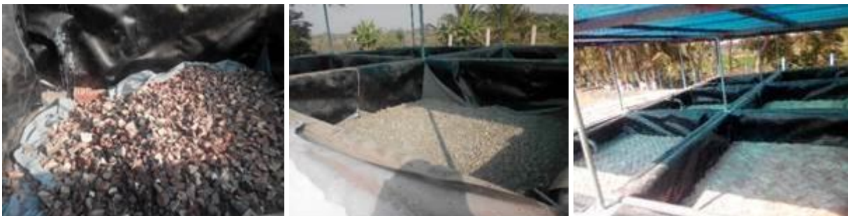
Figure 3. 12 Distribution of filter bed materials in unplanted sludge drying bed.
