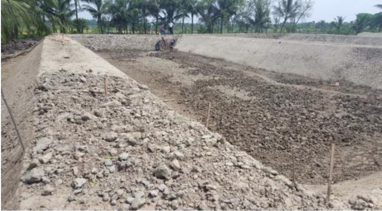
Figure 5. 1 Earthen embankment at Khulna FSTP
