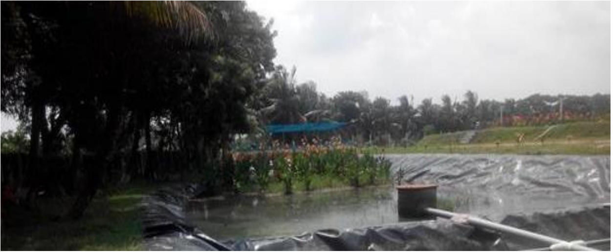
Figure 5. 10 Constructed wetland no. 7 (horizontal subsurface flow) at Khulna FSTP in wet season
