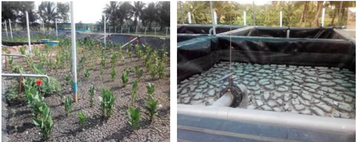
Figure 5. 7 Dried sludge in planted CW and unplanted sludge drying bed.
