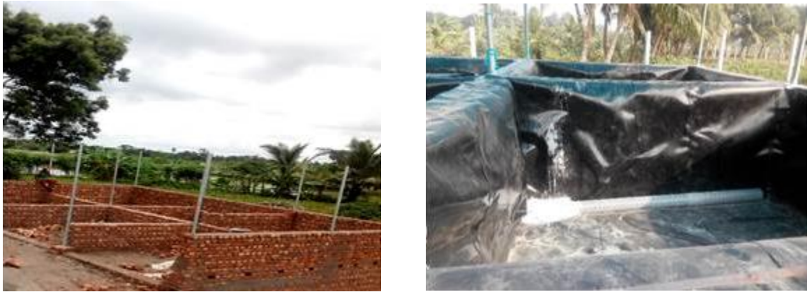
Figure 3. 11 Construction phase of unplanted sludge drying bed at Khulna FSTP.
