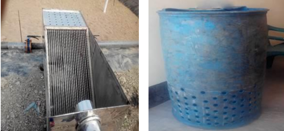
Figure 5. 4 Manual screening (SS304) for VF-CWs and locally made plastic container screen for drying beds
