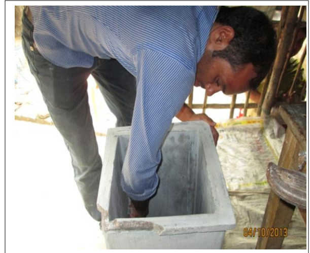
Figure 05 Removing lime from filter unit, March, 2014. Kaligonj
