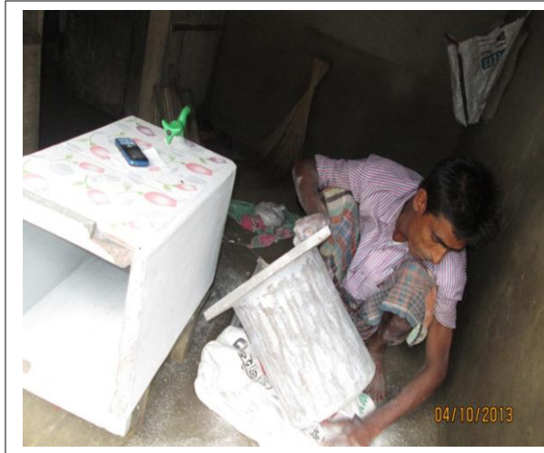
Figure 05 Removing lime from filter unit, March, 2014. Kaligonj
