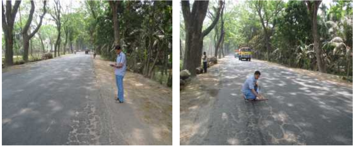
Figure 3.3: Visual Surveys on Test road
