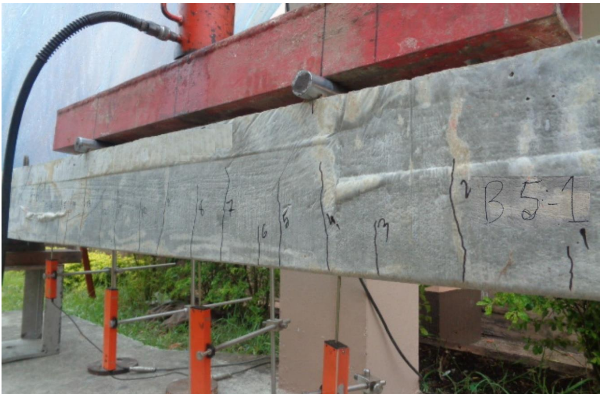
Figure A-14: Crack pattern for preloading (B5-1)
