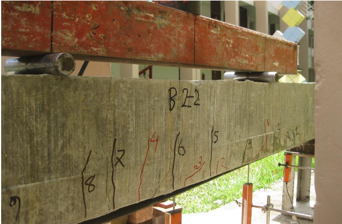
Figure 5.10: Failure mode of beam strengthened with steel plate (B2-2)
