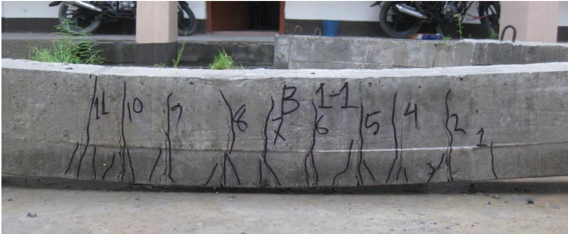
Figure 5.2: Failure mode and crack pattern of control beam (B1-1)
