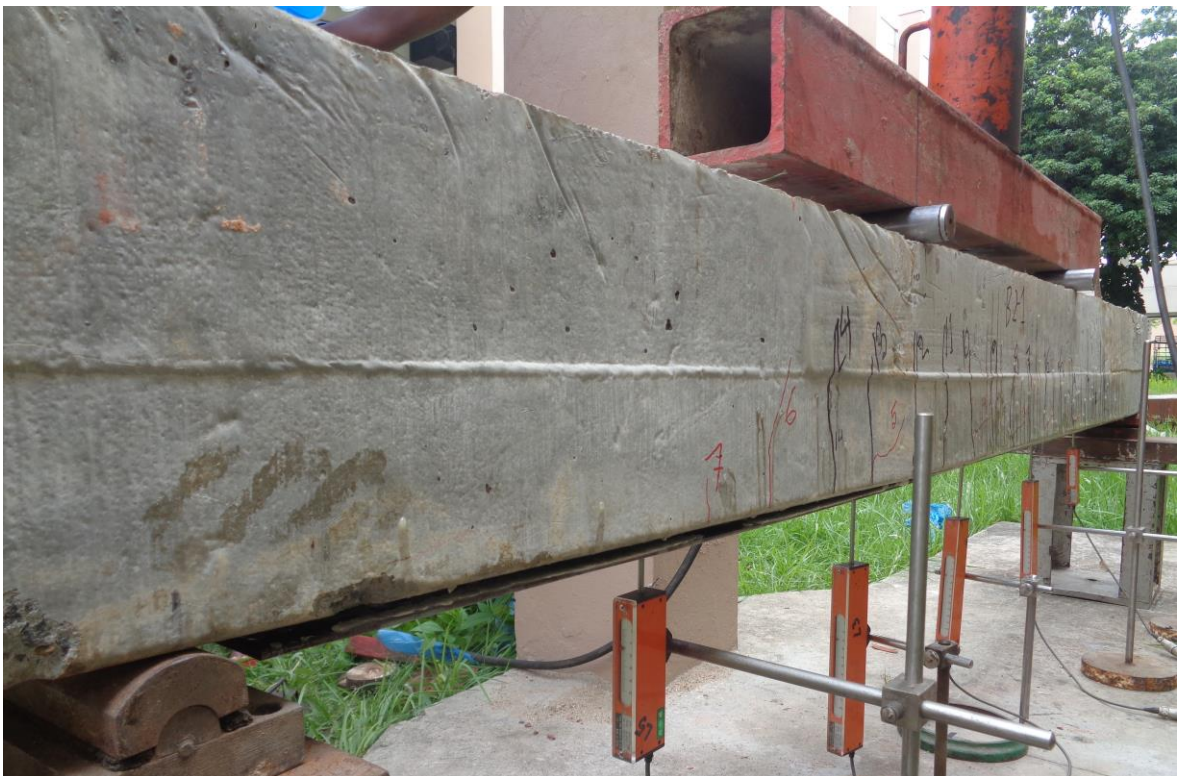
Figure 5.8: Failure mode of beam strengthened with steel plate (B2-1)
