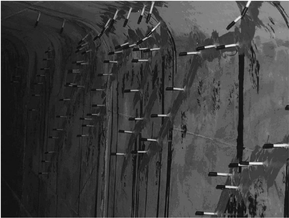
Figure 2.1: Structure prepared for epoxy injection through the ports shown
