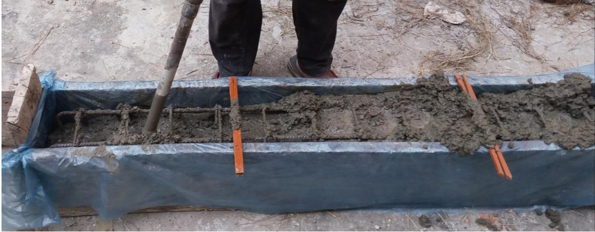
Figure 4.4: Casting of reinforced concrete beams
