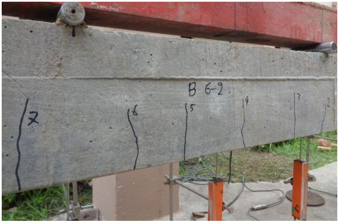
Figure A-20: Crack pattern for preloading (B6-2)
