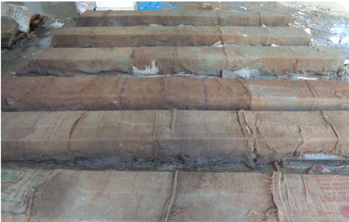
Figure 4.5: Curing of reinforced concrete beams
