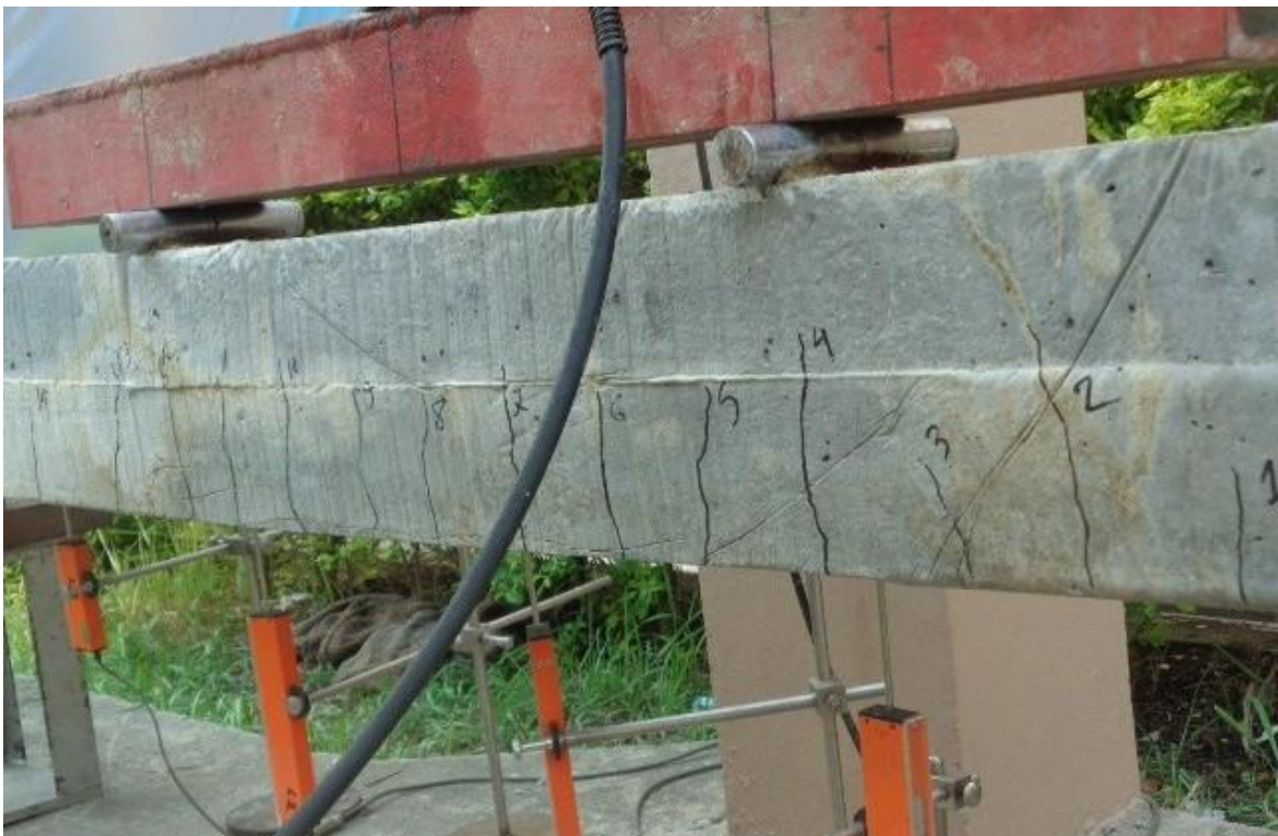
Figure A-6: Crack pattern for preloading (B3-1)
