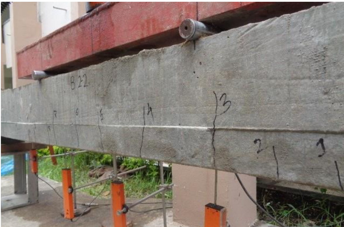
Figure A-4: Crack pattern for preloading (B2-2)
