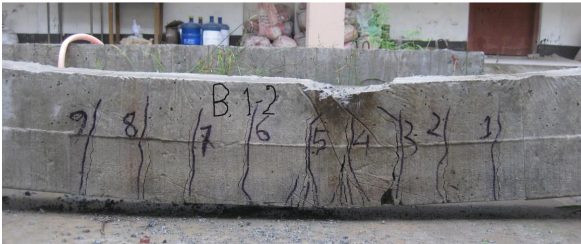
Figure 5.4: Failure mode and crack pattern of control beam (B1-2)
