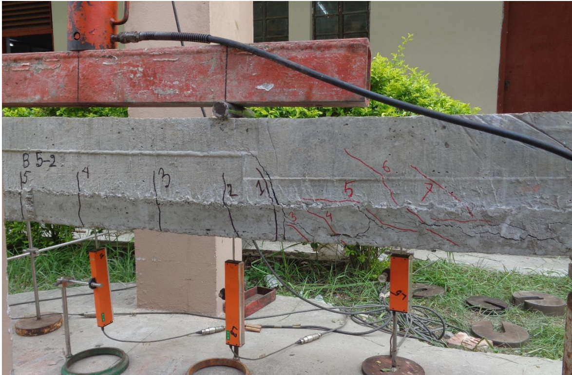
Figure 5.22: Failure mode of beam strengthened with steel angles (B5-2)
