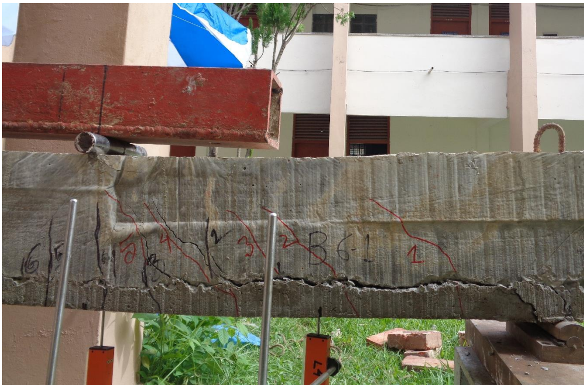
Figure 5.24: Failure mode of beam strengthened with steel bars (B6-1)
