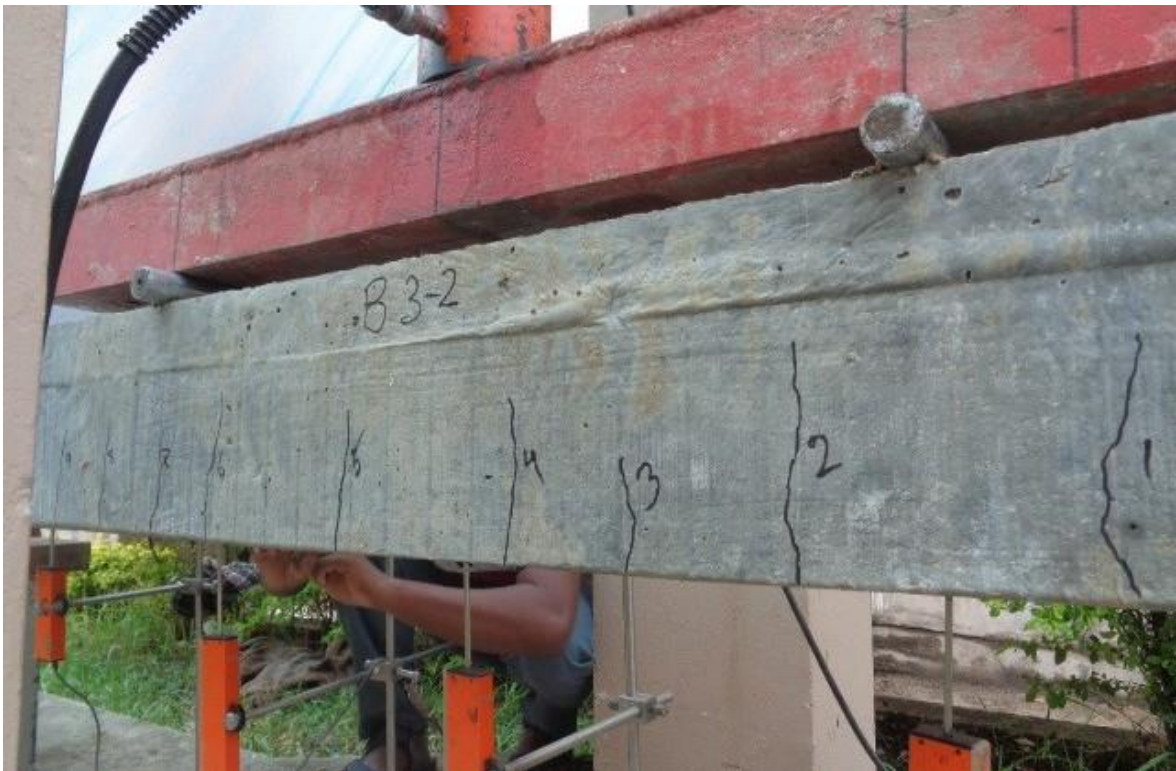
Figure A-8: Crack pattern for preloading (B3-2)
