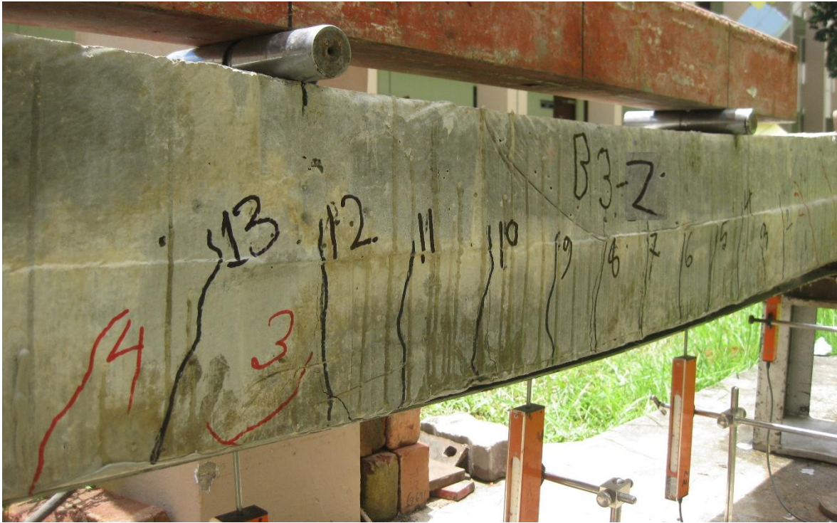
Figure 5.14: Failure mode of beam strengthened with steel plate and bolts (B3-2)
