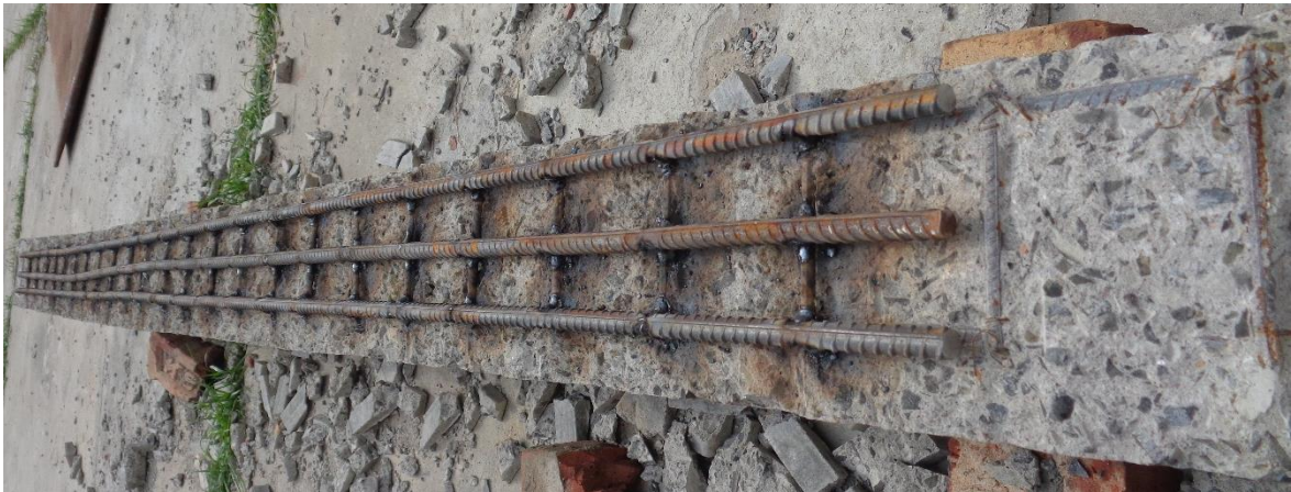
Figure 4.14: Strengthening with external steel bars
