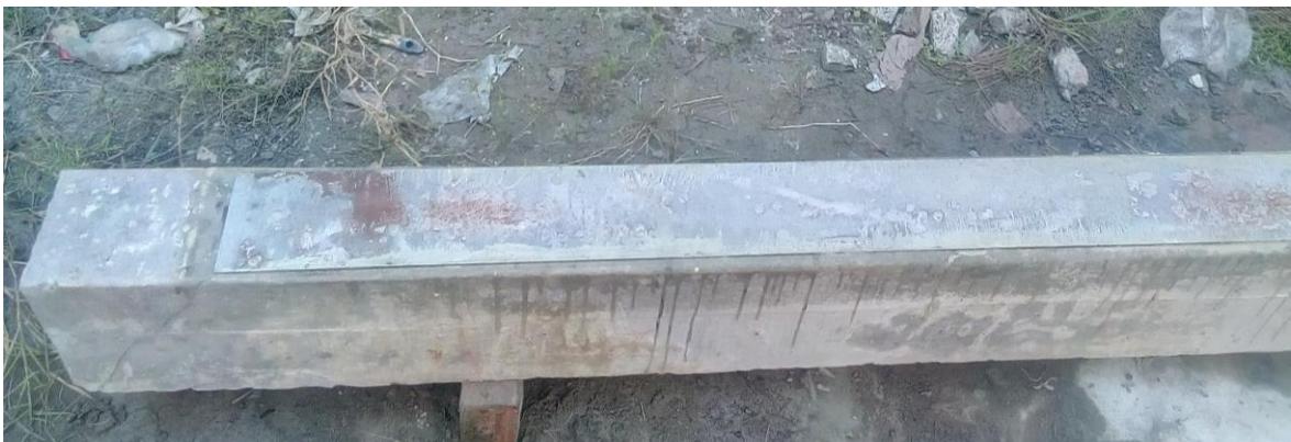
Figure 4.10: Strengthening with external steel plate
