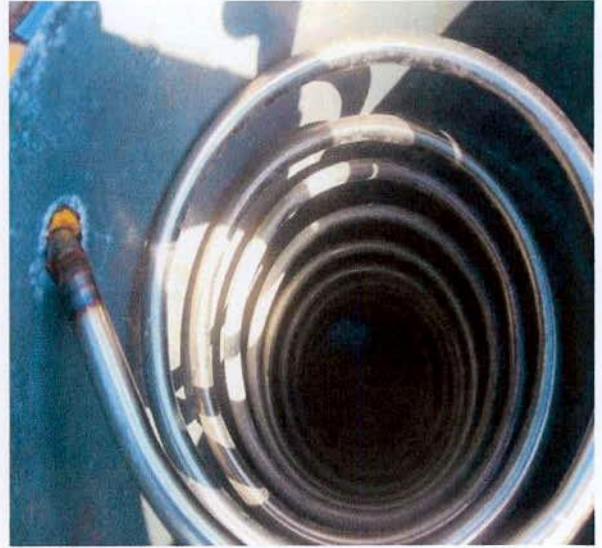
Figure 3.10: Inside view of Condenser coil container
