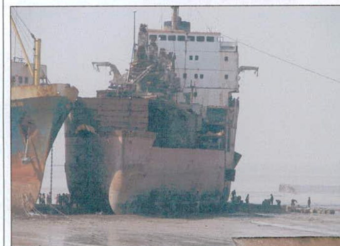
Picture -3 : Dismantling starts from the nose
