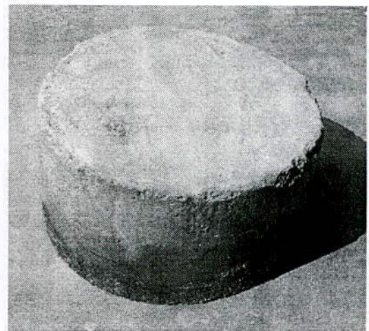
Fig. 3.16 RCC footing
