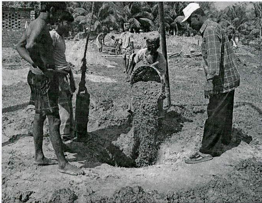
Figure 4.5 Pouring of mixed granular materials.
