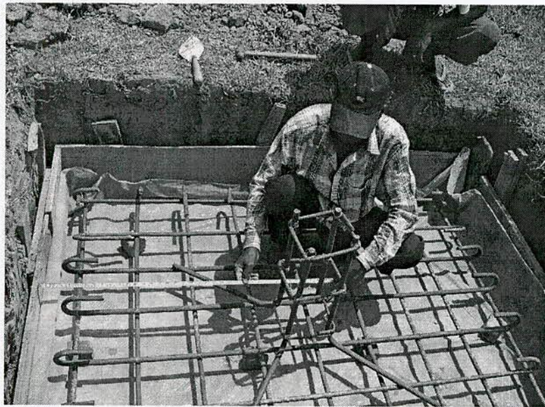
Figure 4.10 Construction of footing on Rammed Aggregate Piers treated ground.
