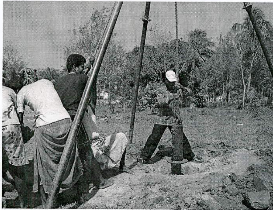
Figure 4.6 Compaction of granular materials.
