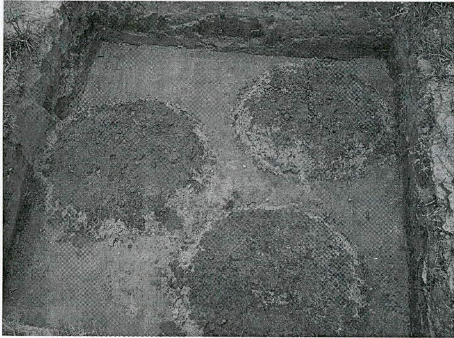
Figure 4.9 Completed Rammed Aggregate Piers in the ground.
