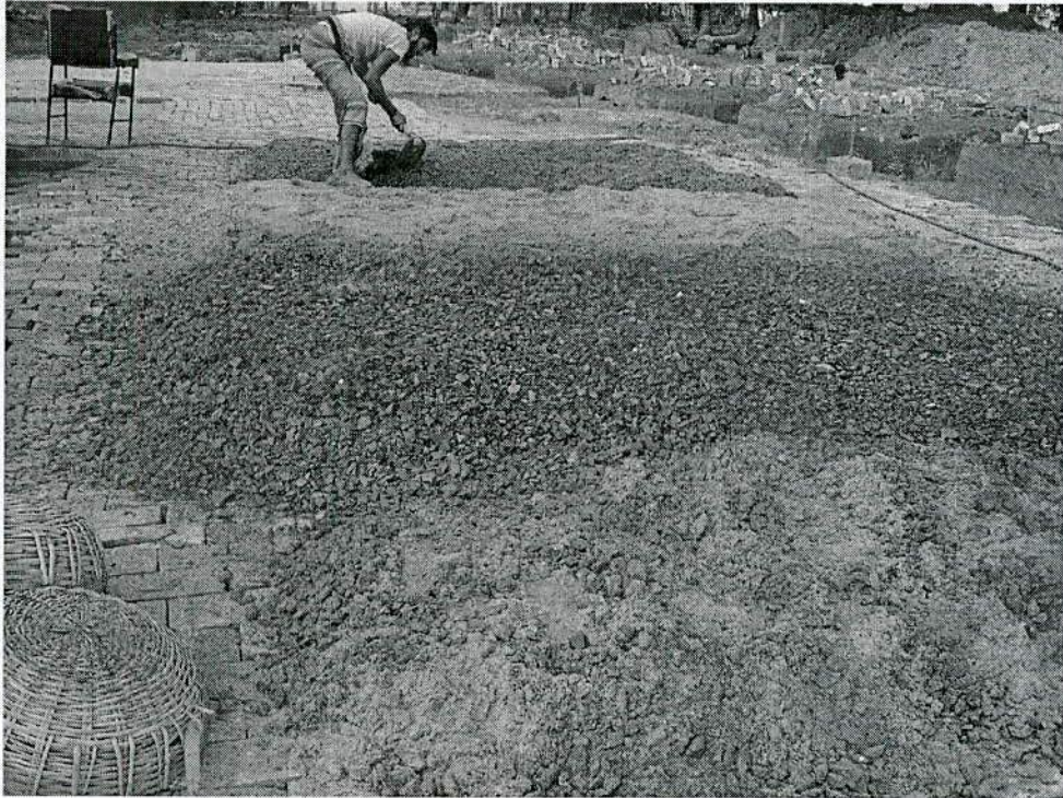
Figure 3.8 Granular materials used in Rammed Aggregate Pier construction.
