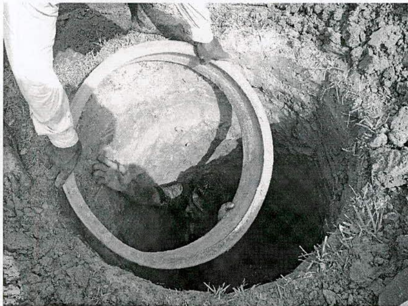
Figure 4.4 Placement of casing during the excavation hole for RAP construction.
