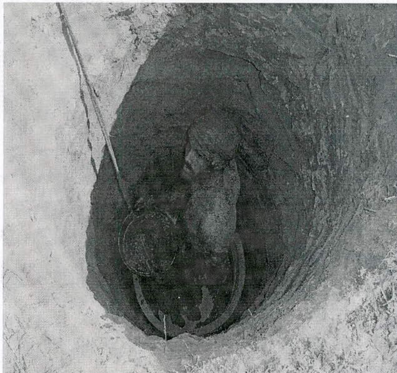
Figure 4.2 Excavation of hole to install RAPs.
