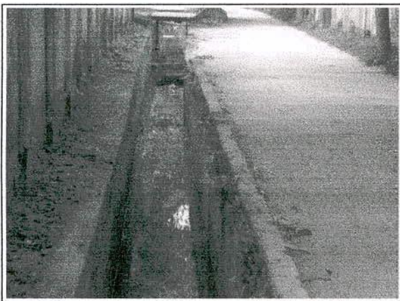
(C) Drain beside road (Bhola Pourashava).
