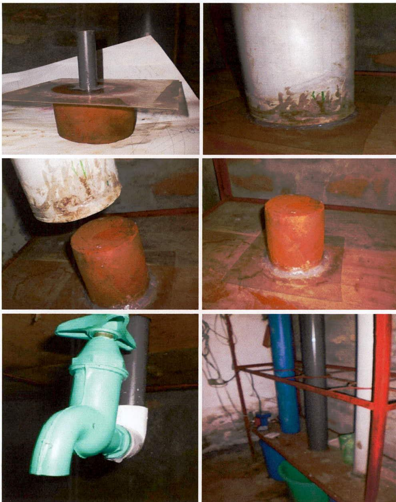
Fig: 3-7 Setup of CMBR after clogging
