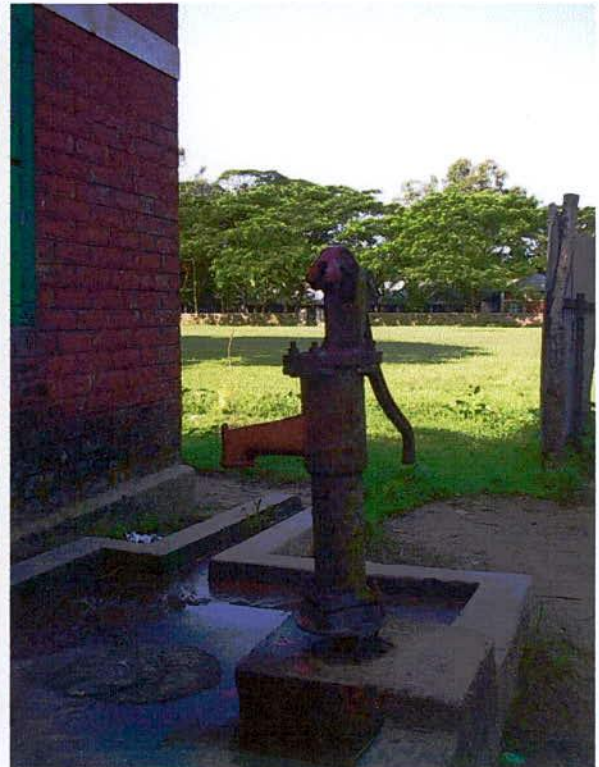
Fig: 2-20 Greywater is discharged to surface drain from tube-well spot
