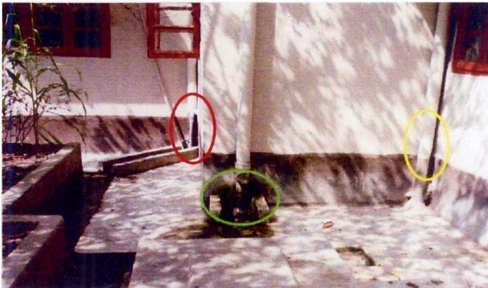
Fig: 2-17 Greywater Scenario for urban areas: a house with 3 outlets, red-color from kitchen, green-color from bathrooms and yellow-color from toilets
