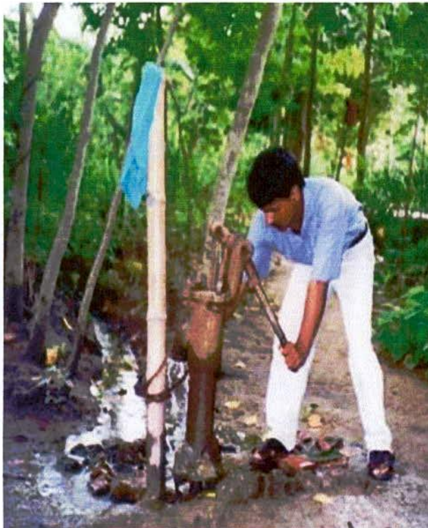
Fig: 2-20 Greywater is discharged to surface drain from tube-well spot
