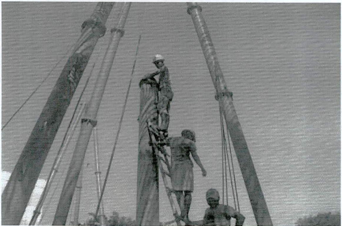
Fig. 4.5 Pouring the granular material into the created hole.
