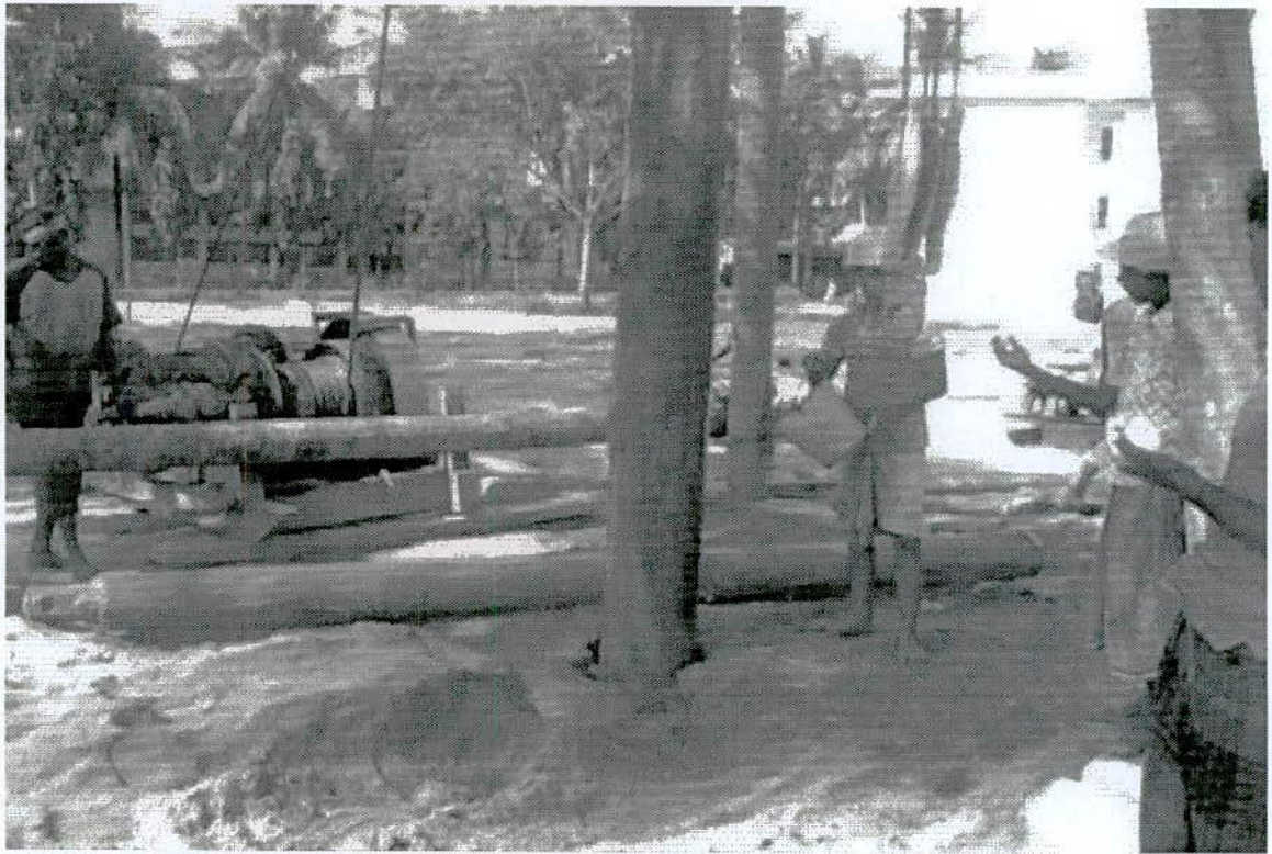
Fig. 4.4 Lifting of 300mm diameter steel pipe
