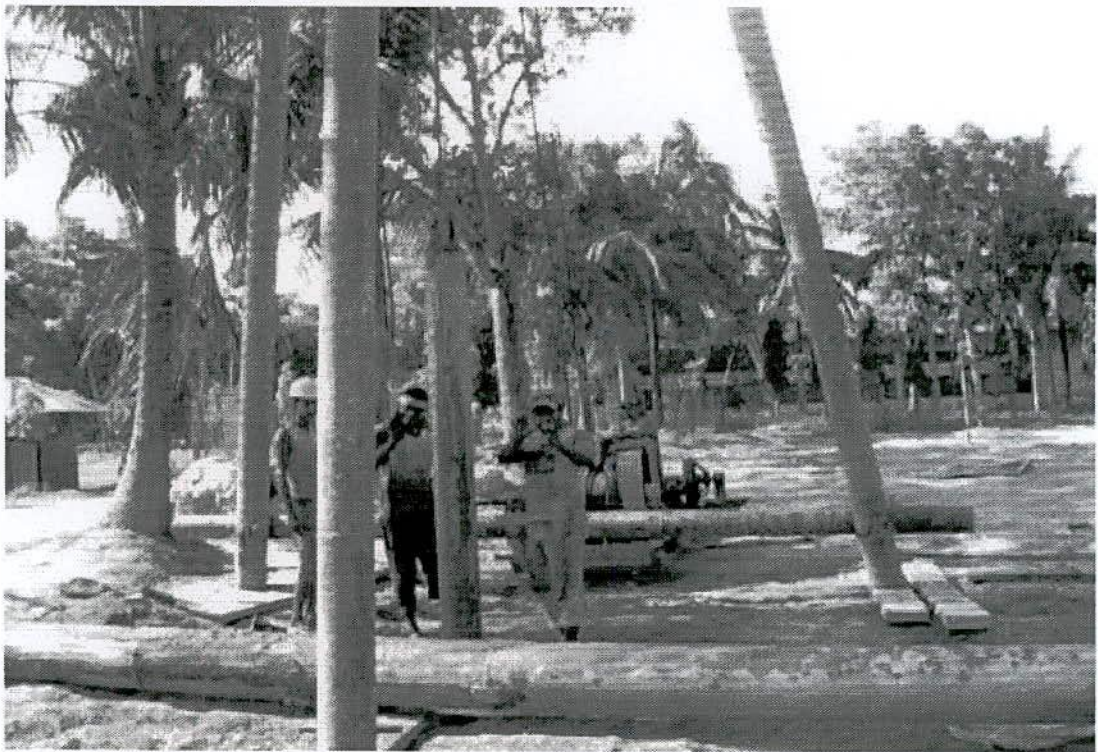
Fig. 4.2 Investigation field during construction of granular piles
