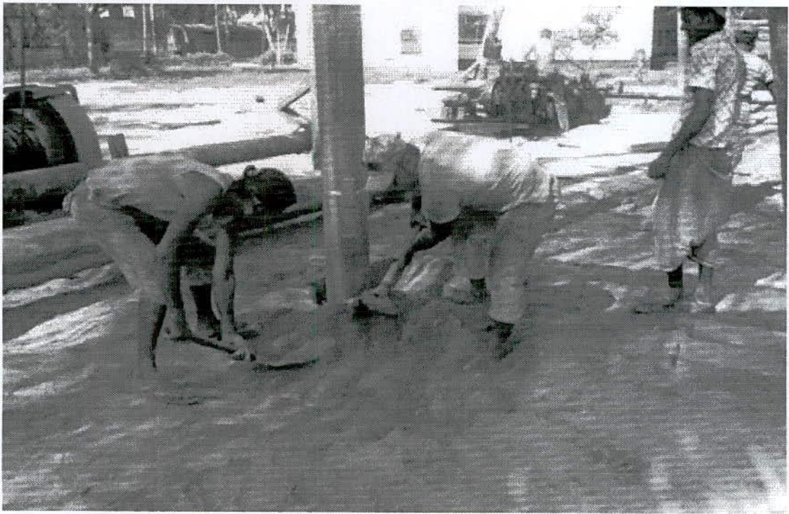
Fig. 4.6 Compacting the granular materials inside the ground.
