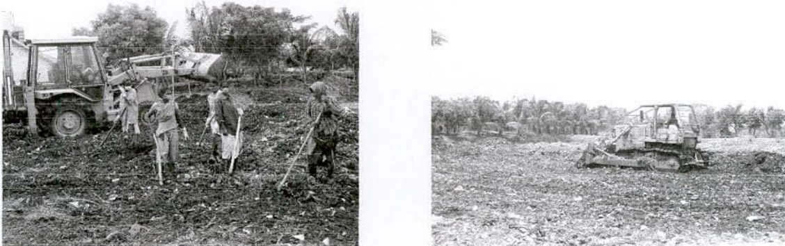
Figure 4.5 Waste spreading and compaction operation at the PSSL
