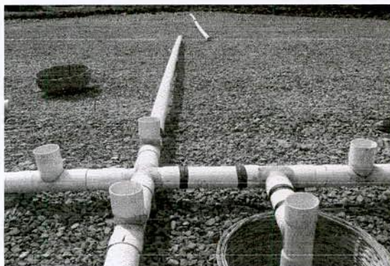
Figure 4.17 Top covering of PSSL with Gas Ventilation Pipe
