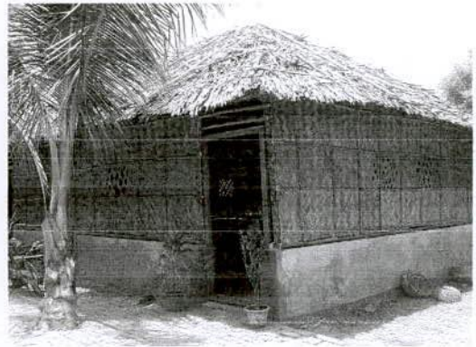
Figure 4.3 Site office beside the PSSL
