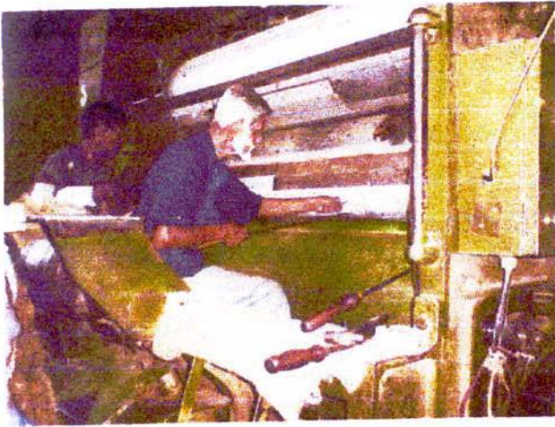
Picture-1: Fitters are fitting staves with hand tools.
