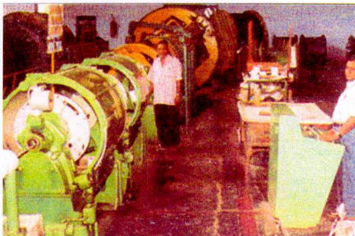
Figure-3.2-7: Main Unit & Core Stranding Machine.
