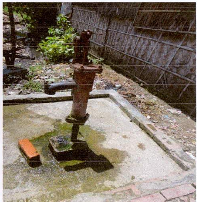
Figure 4.3(B): Unhealthy Drainage system at No-4, Kasem nagor road, Gollamari Dakshin, Khulna.
