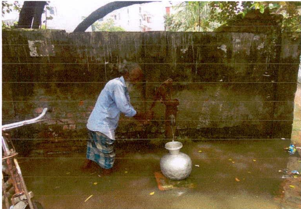
Figure 4.4: Water logging around tube-well at Daroga Para
