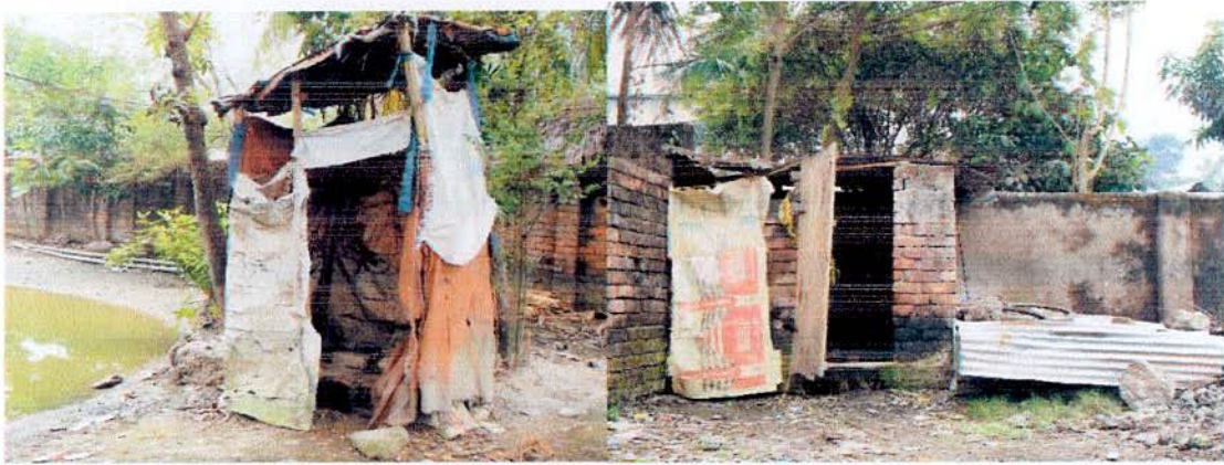
Figure 4.17: Water source and latrine at the same place
