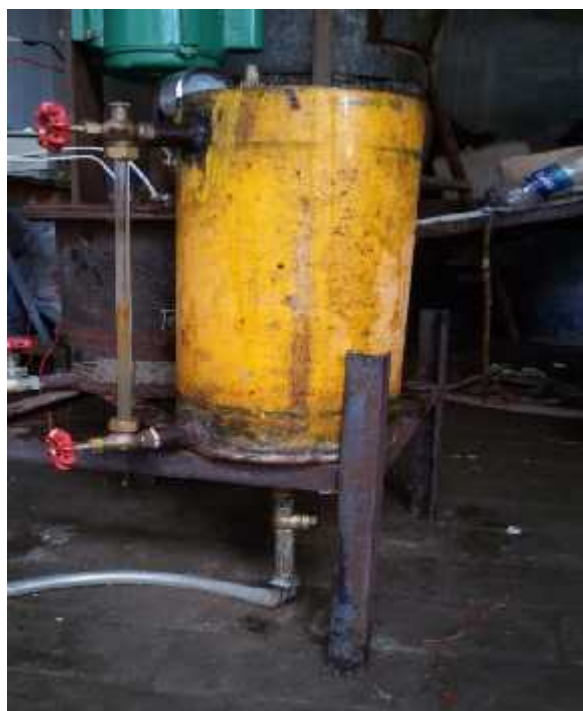
Figure 4.3: Photographic view of Washing vessel and Separator
